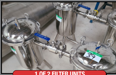
1 OF 2 FILTER UNITS
