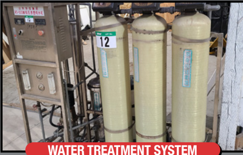
WATER TREATMENT SYSTEM
