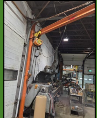
1 OF MANY HOISTS
