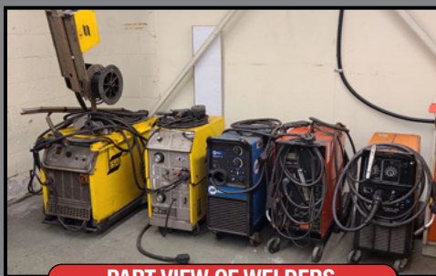
PART VIEW OF WELDERS
